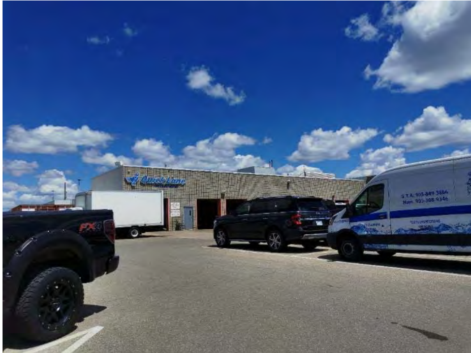
Photo 17: The property located at 570 Trafalgar Road, east adjacent, facing northeast.
