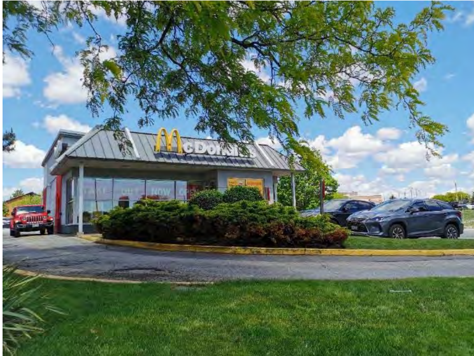
Photo 1: Frontage of the Site at 227 Cross Avenue, facing north.
