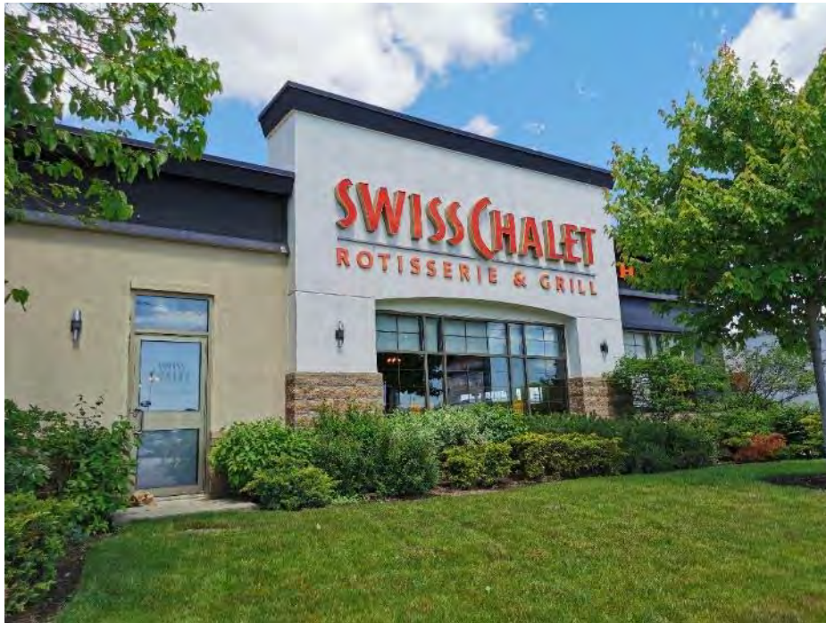
Photo 2: Frontage of the Site at 217 Cross Avenue, facing north.
