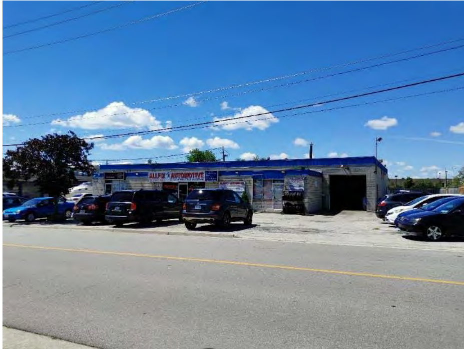
Photo 13: The property located at 570 Argus Road, approximately 20 m west, facing west.
