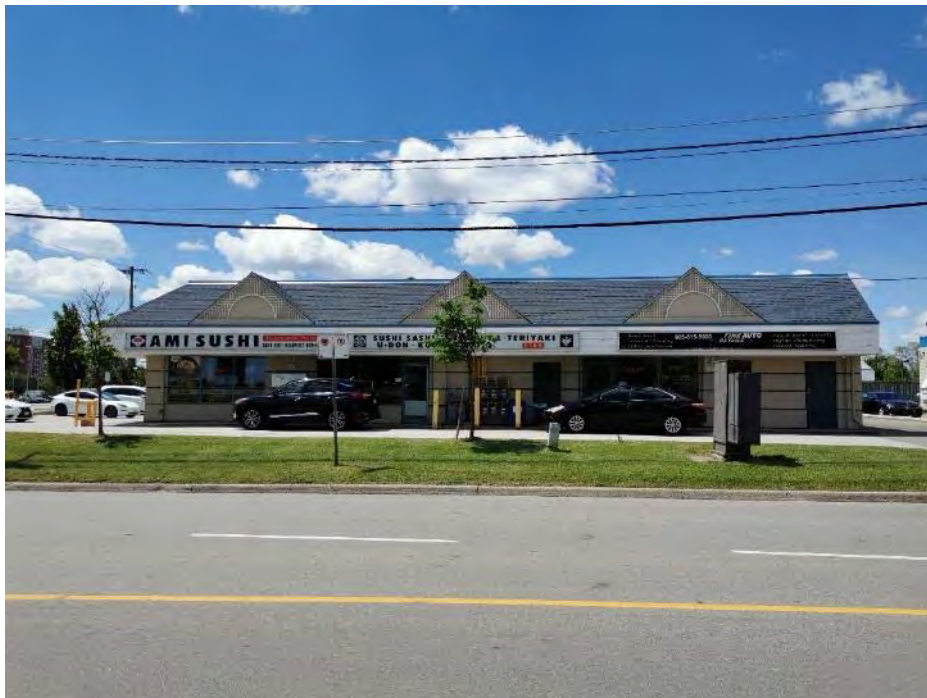
Photo 14: The property located at 568 Argus Road, approximately 20 m west, facing west.
